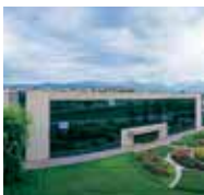
The New Factory
